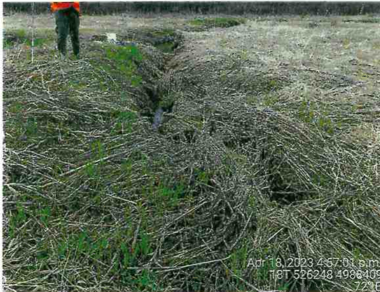
Photo 10: Station 2, looking downstream from near its upstream end (April 18, 2023)
